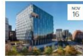
AIA UK BUILDING TOUR SERIES 2023 - US EMBASSY BY KIERAN TIMBERLAKE
